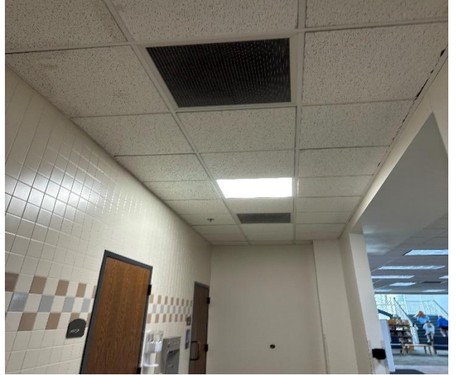
Photo 4) 1 st Floor Bathroom Entry - Overview
