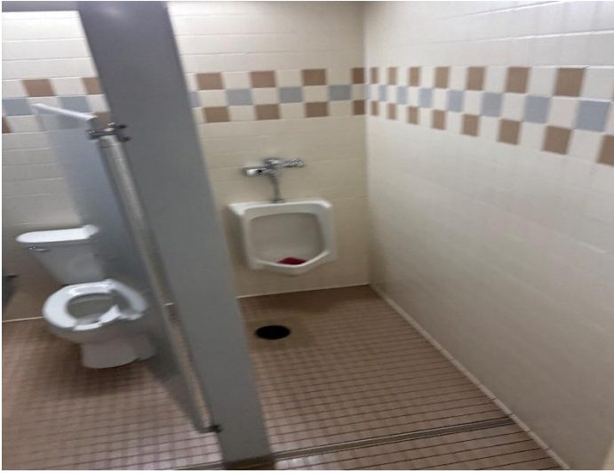
Photo 1) 3 rd Floor Men's Bathroom (Representative of all Bathrooms)
