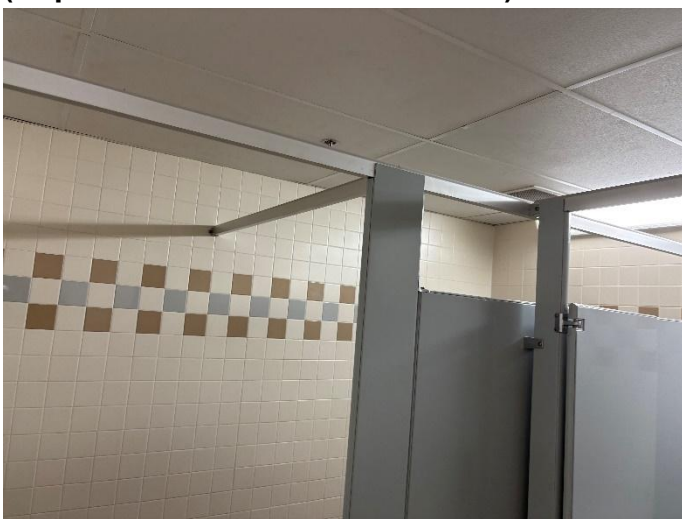
Photo 3) 3 rd Floor Men's Bathroom (Representative of all Bathrooms)
